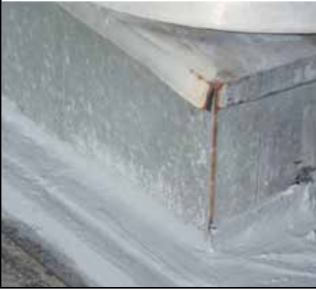
Polyprene® around roof curb.
