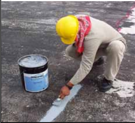
Polyprene fills gaps in cracks on concrete roof.
