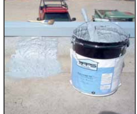
Seals wall flashing and field seams on modified membrane.
