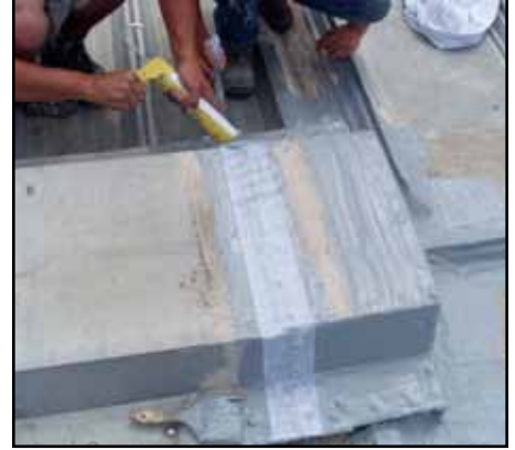
Caulk tube application for precise placement.
