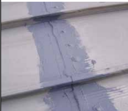
Polyprene forms to the shape of the roof and clings to seams.
