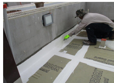
Insulation/Cover Board Installation
