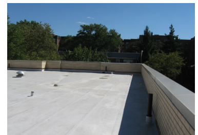
Typical Built Up Finished Roof
