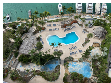
Vegetated Roof Deck
