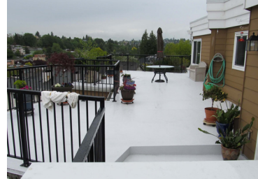
Carports - Roof Decks
