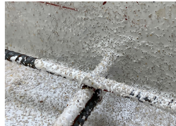
Re-bar Encapsulation
